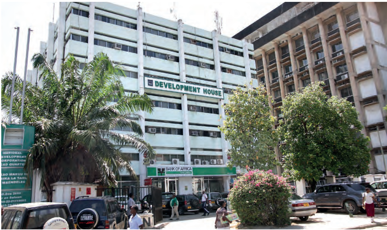
Outside view of BOA in Tanzania Head Office, in Dar es Salaam.
