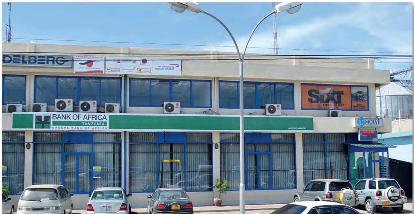
Outside view of Airport Branch.
