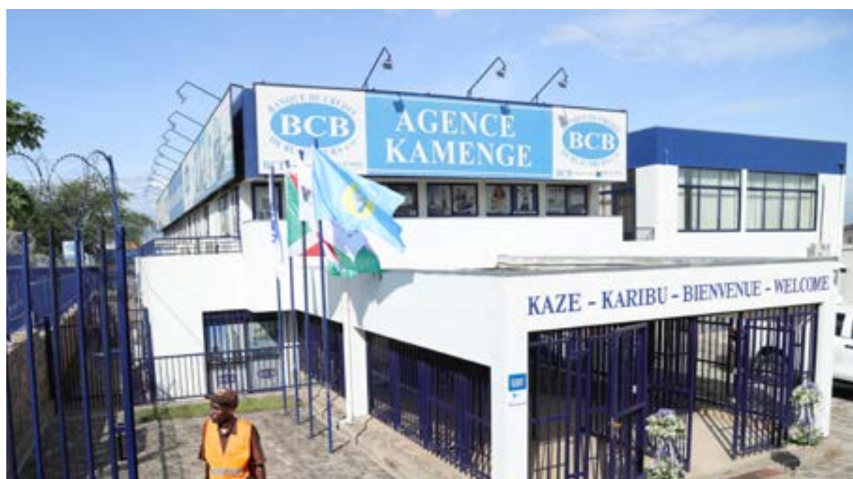
View of Kamenge Branch's customer entrance
