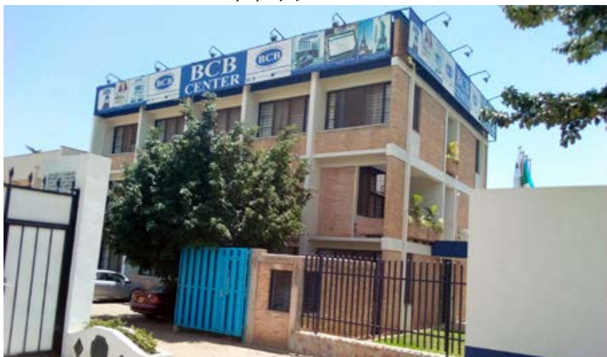
View of BCB Center building
